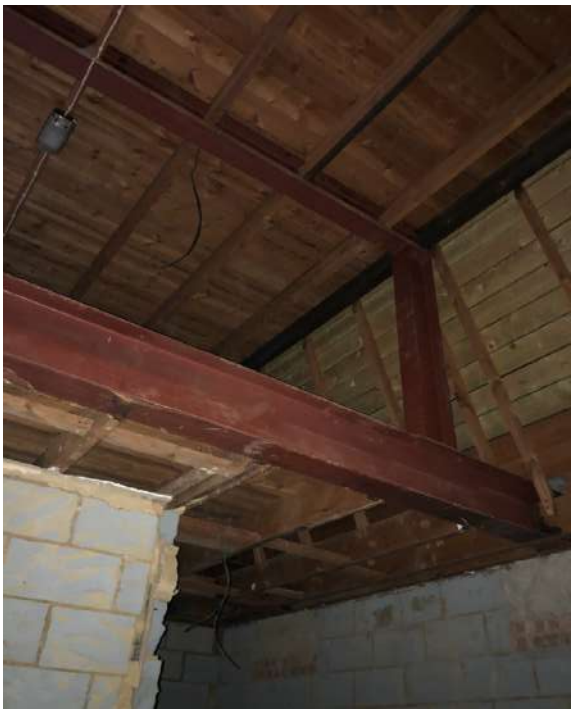
General roof structure - plantroom floor will be created between beams by Builder
