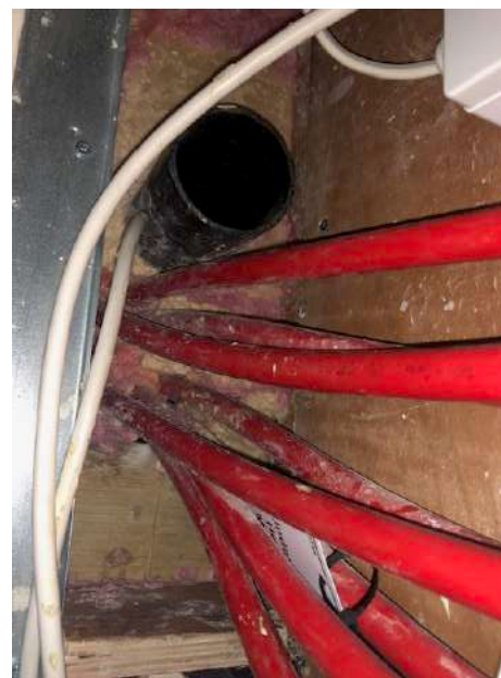
REF: 160620-6 Fire stopping: There is no vertical fire stopping within the main stairwell and as a consequence the whole house is sprinklered. Building Control to confirm that no additional fire stopping is required within the risers
