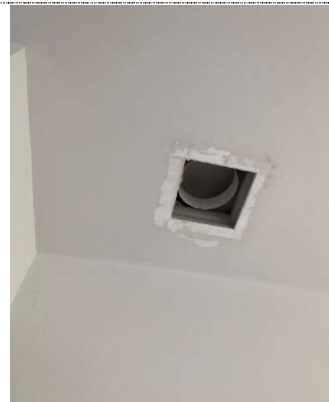
REF: 160620-8 Gas fire natural ventilation How is the duct connected to the external air brick? Does it penetrate the cavity & physically connect by a plenum box? See also REF: 300620-9
